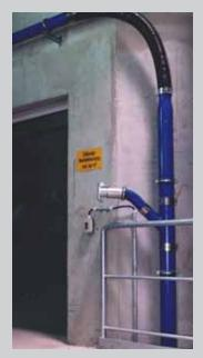
Piping system with suction inlet valve DN 50 (2") for the cleaning of machinery and floors on the different levels
