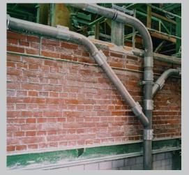
Pipework systems bring the suction power to the areas where vacuum cleaning is required. Set-up time is not required. The operators can immediately start with the cleaning work.
