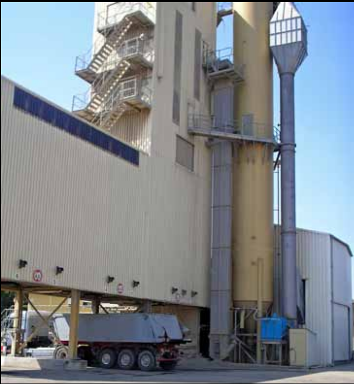
Vacuum cleaning of dust in a mixing plant for additives.
