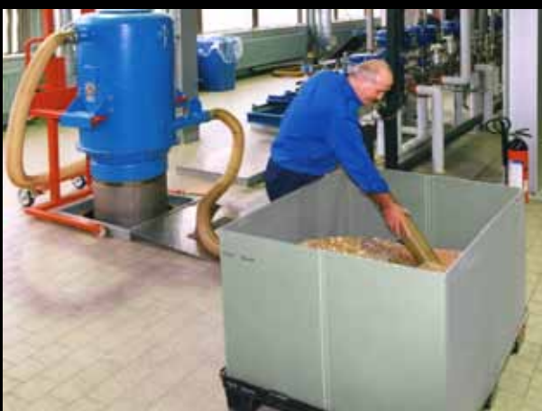
Vacuum conveying of blended spices to the production process
