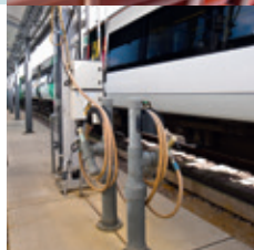
MULTIRAIL® SandPiper Train & tram sandbox filling systems
